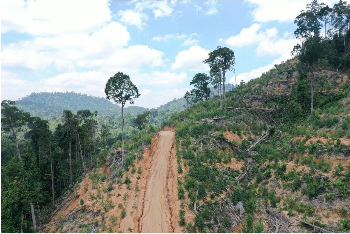
Figure 20. Clearing within PT Wana Hijau Pesagan, image from February 2021.
